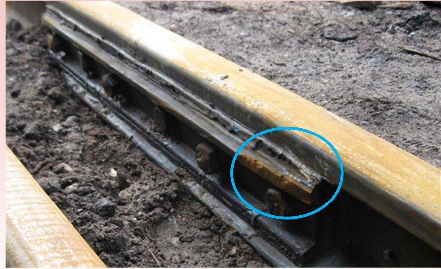
Low-side IJ also shows receiving end batter
