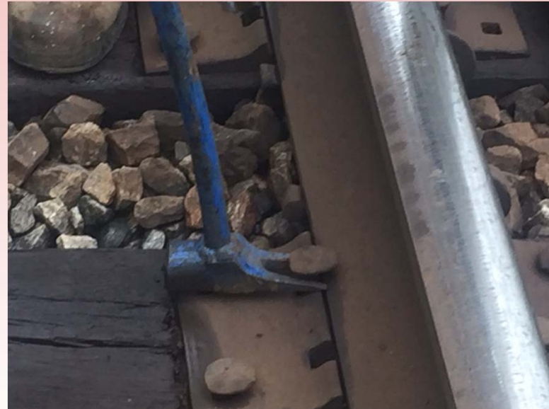
Step 2: Attempt to pry the spike up. If it is broken, the top half will pull out.
