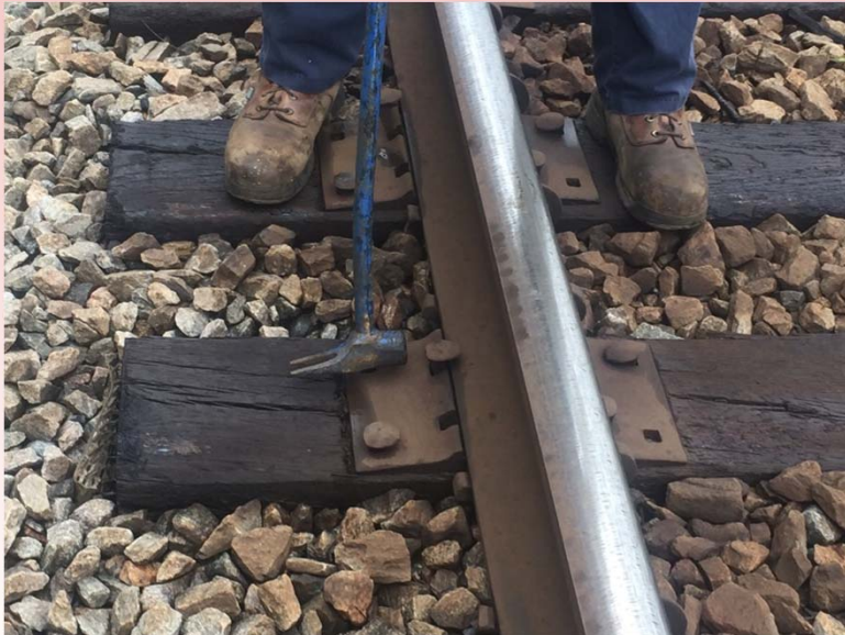
Step 1: Hit the heel of the spike to see if it is loose or makes an unusual sound.
